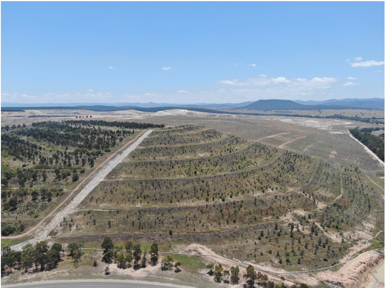
Photo taken December 2025 showing rehabilitation progression of the Southern Rehab
